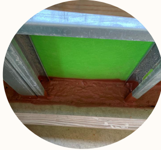
Edge-of-slab joint
